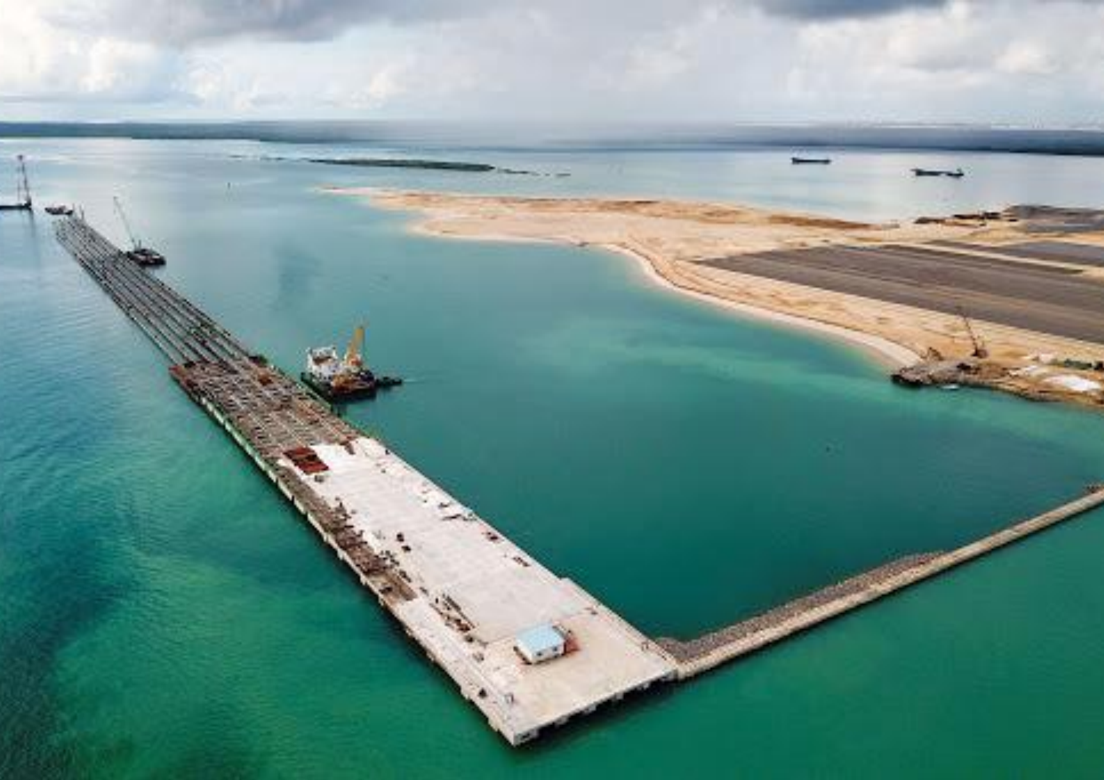
img_3 : LAPSSET project under progress
