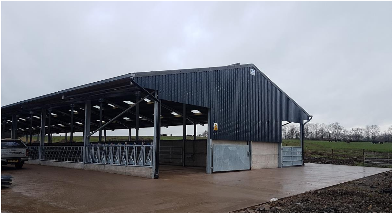
Fig: 3 – Problem - Despite any location a dairy farm is an engineering solution
