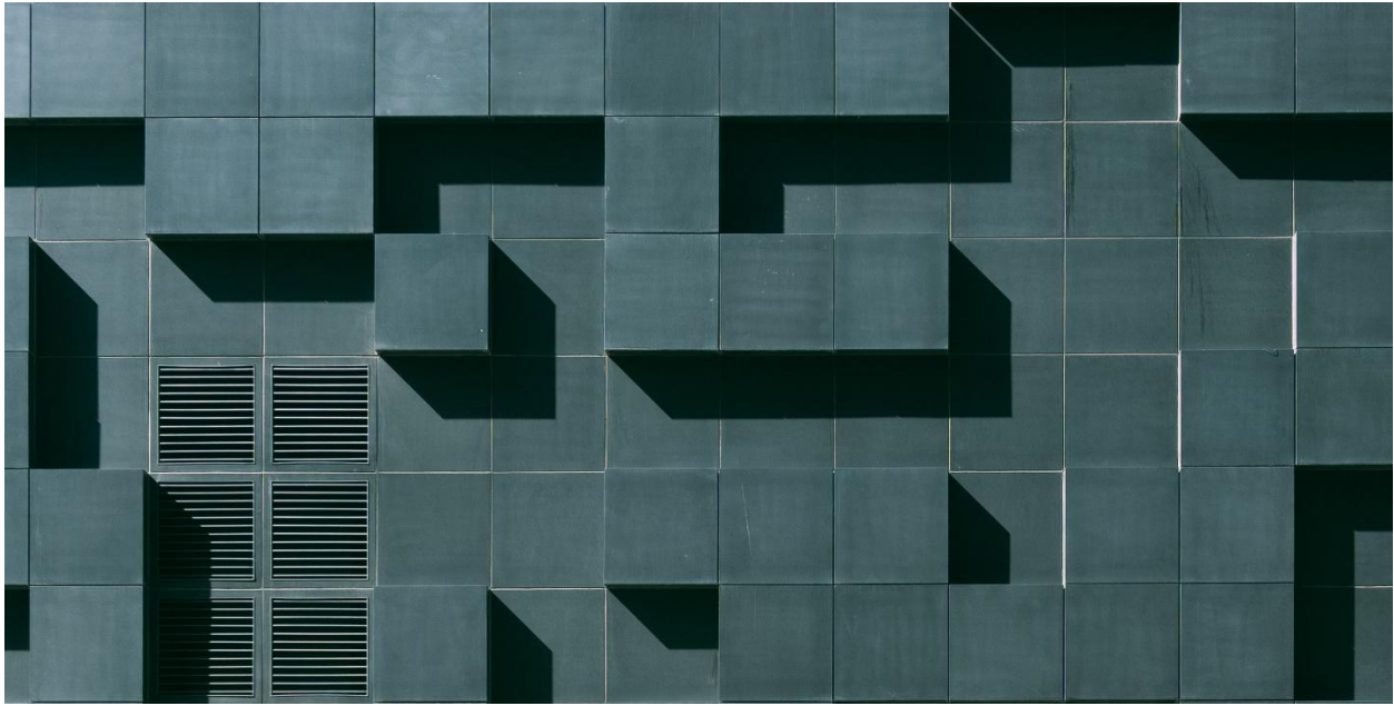
Fig: 1 – Squares as an element on a building façade – An illustration
