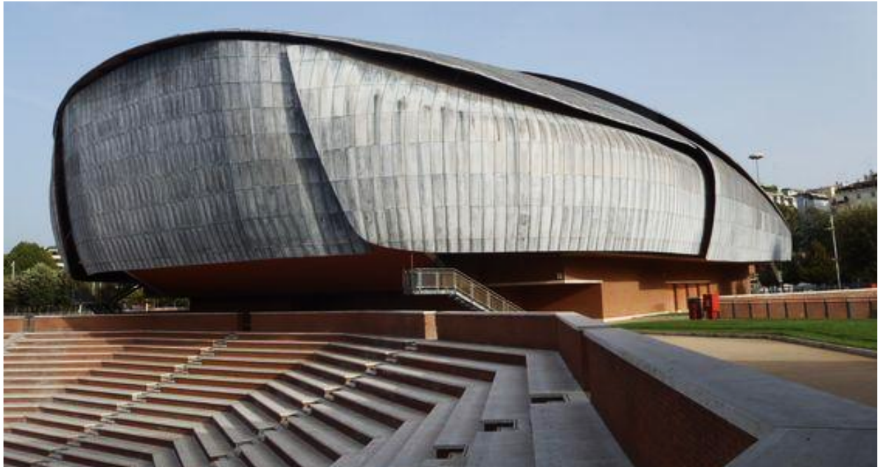
Fig: 2 - This music auditorium was built by incorporating the ruins of an ancient Rome villa and restoring it to blend seamlessly with the design of the complex. (Credits: SCE PROJECT – Cristiano Bendinelli)
