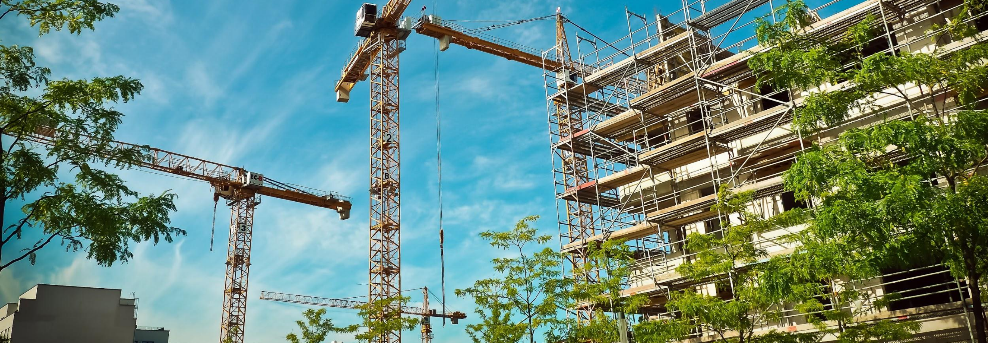
Img_1: Modern day construction site.
