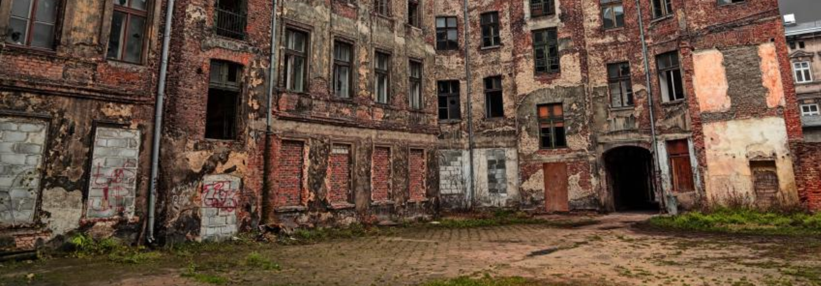
Img_3: State of abandoned buildings.
