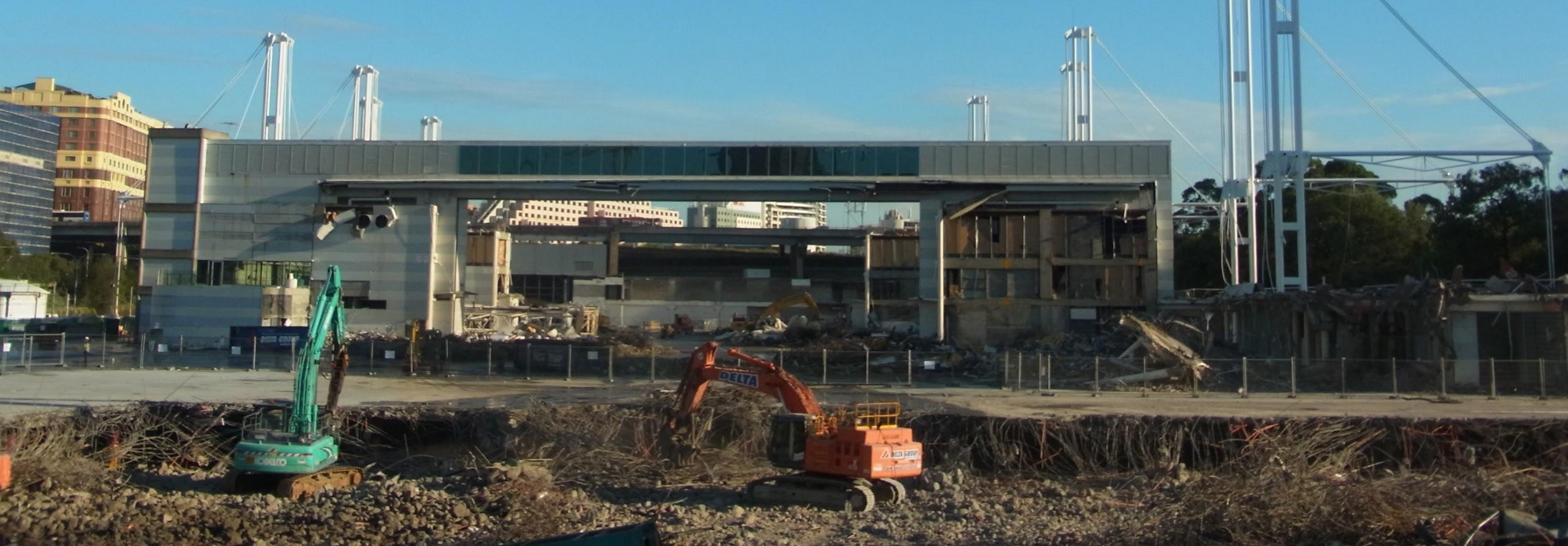
Img_2: Demolition of Sydney Convention and Exhibition Center designed by Phillip Cox in March 2014.
