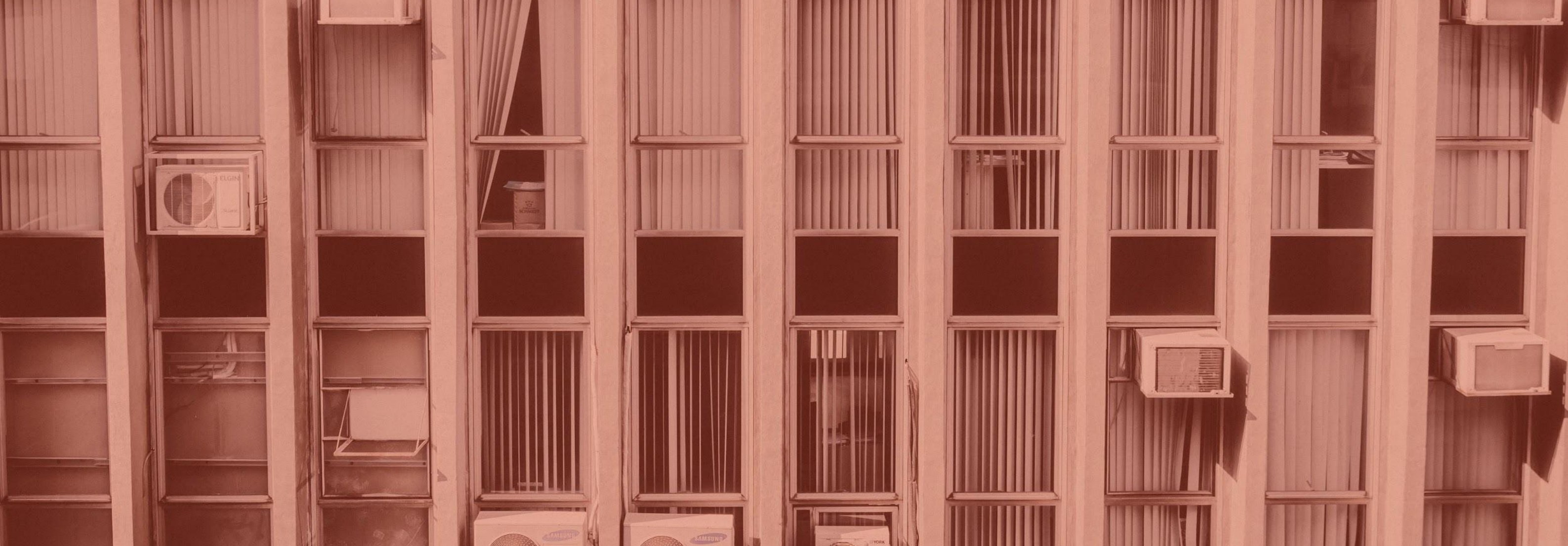
Img_3: Building facade that has surrendered to external cooling methods.
